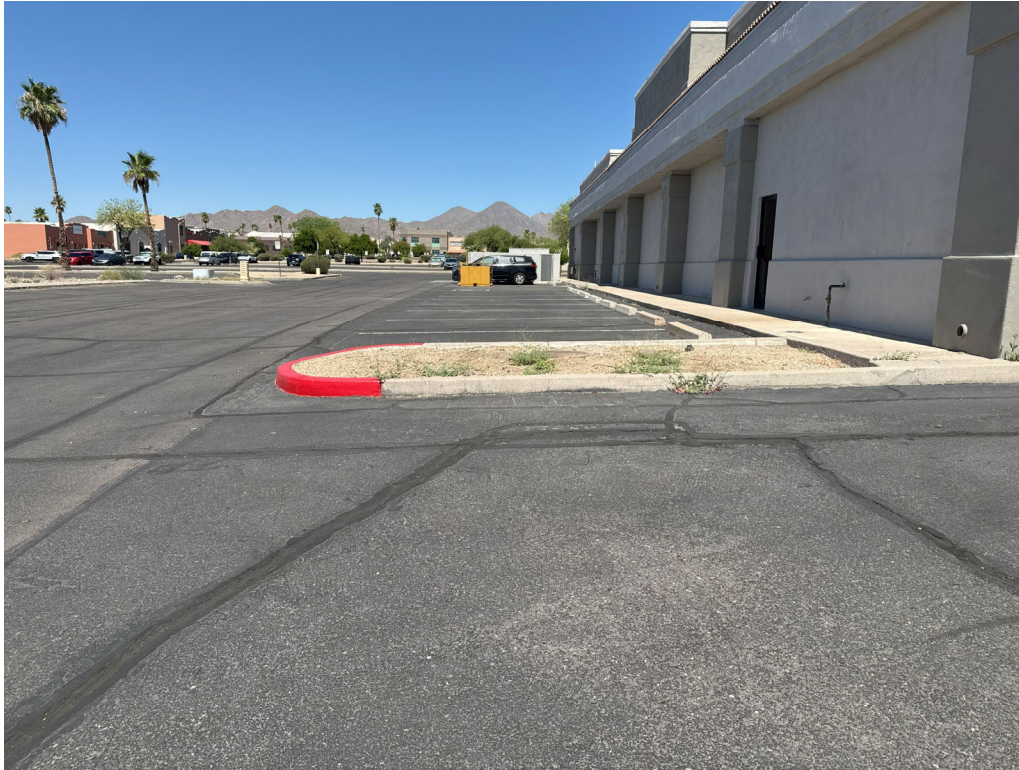
Photo of rear of building looking west.
