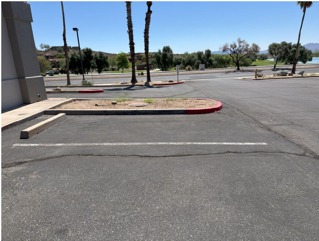
Photo of rear of building looking east. This is the island that will be removed for the drive thru lane.
