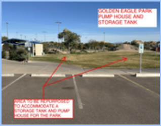
GOLDEN EAGLE PARK - PUMP HOUSE STORAGE TANK SITE
