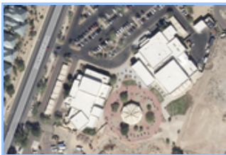
Library-Museum-Community Center Air Handlers.jpg
