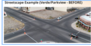
Verde-Parkview Intersection Before.JPG
