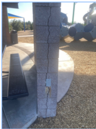
Structural Cracking
