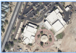
Library-Museum-Community Center Air Handlers.jpg
