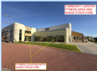
COMMUNITY CENTER - FITNESS AREA - SHADE STRUCTURE
